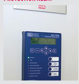
Protection relays are offered for grid-tie and Energy Conversion Systems (ECS).
